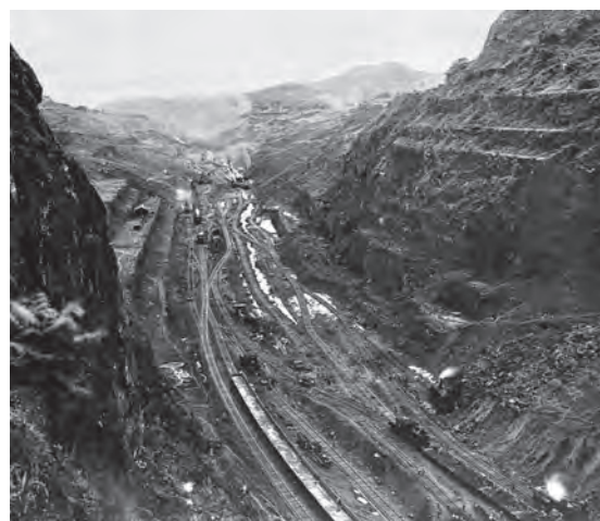
Fig. 2. The Culebra Cut during the American excavations, looking towards the northwest. The steep rock face cut into Gold Hill is on the right, and the lower slopes beyond would subsequently further degrade into the West and East Culebra Slides. (Historical photographs of the American excavations are from the archives of the National Academy of Sciences in Washington.)
