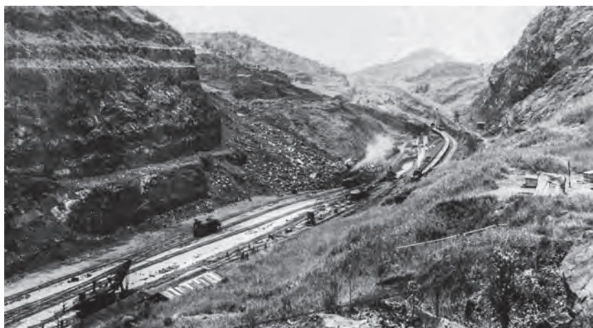
Fig. 8. An early stage of development of the large Cucaracha Slide. Most of the slide debris consists of Cucaracha clay, but the broken rock in the centre of the view is largely volcanic material from the adjacent face of Gold Hill.
