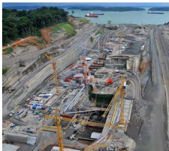
Fig. 17. An early stage of construction of the Agua Clara Locks, with the excavations bounded by steep faces cut into stable Palaeogene sedimentary rocks. (Photo by Panama Canal Authority.)
