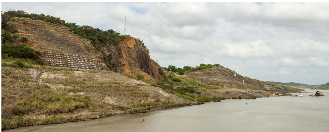
Fig. 13. On the left the anchored wall that has stabilized its rock buttress of Zion Hill after it was seen to be creeping over underlying clay. To its right, the West Culebra Slide has been cut to a much lower profile and is now largely stable, though a floating dredger was working at its toe when this image was taken in 2012.
