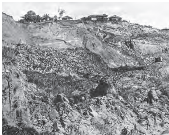
Fig. 10. The West Culebra Slide when successive slices were falling away from the head scarp, thereby undermining and destroying the small hill-top town of Culebra.
