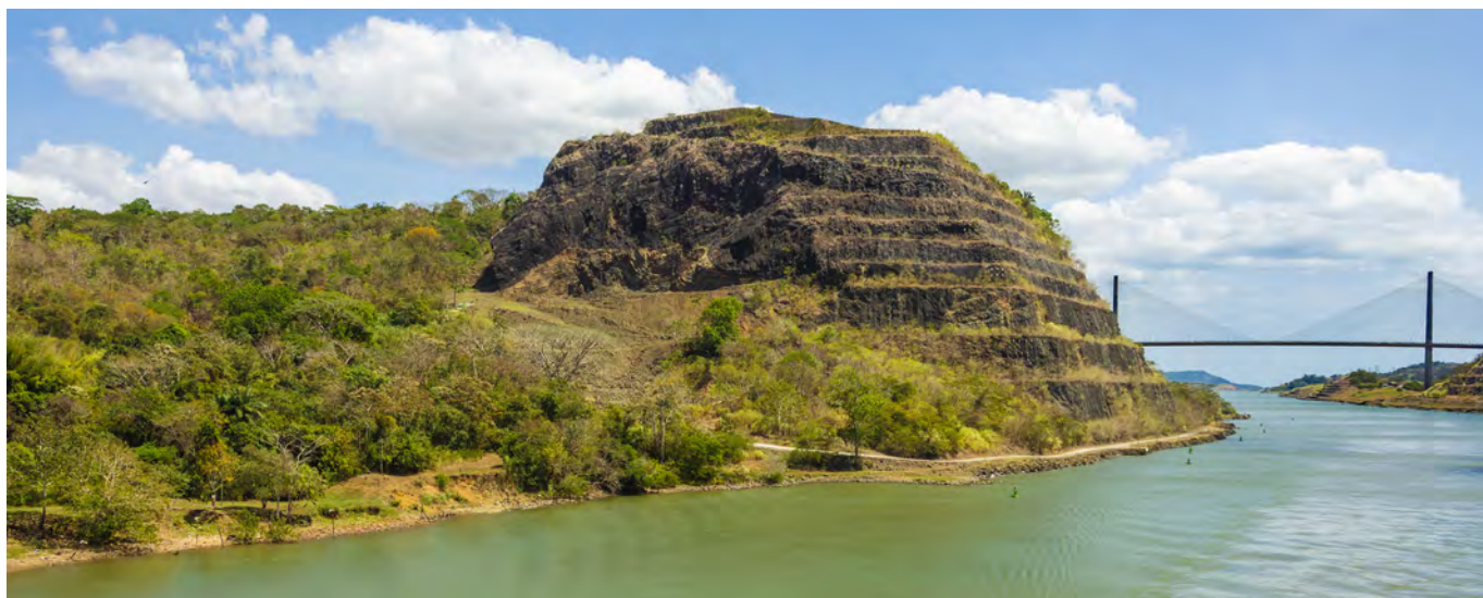
Fig. 12. The Canal's classic view of Gold Hill with the Centennial Bridge beyond. Though the terraced rock face of Gold Hill is the conspicuous feature, the low slopes on the left are actually more remarkable as they are all that is left after removal of most of the very large East Culebra Slide.
