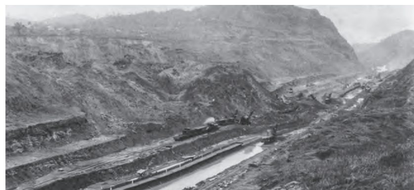
Fig. 9. An early stage of the East Culebra Slide, in 1913, before continued slumping and toe removal left a much lower profile on this bank of the canal.
